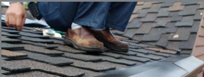
Installation of GutterSheds on gutters built into a roof with very thick shingles
